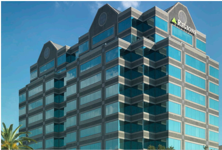
Tower Place in Tampa, Florida, is a Class A high rise office building with on-site bank, café and fitness center
